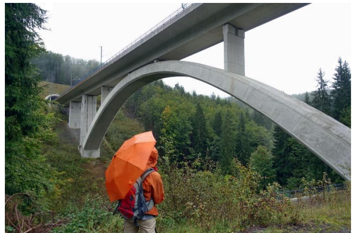
Rehtalbrücke © Ch. Paetzold
